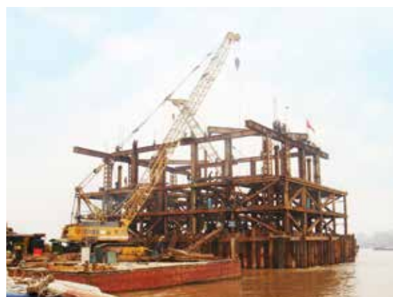
Underwater constructional scaffolding
