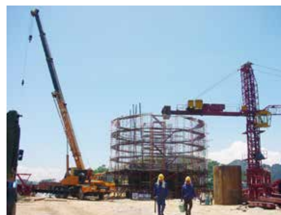
Construction of caisson and abutment for Bai Chay Bridge
