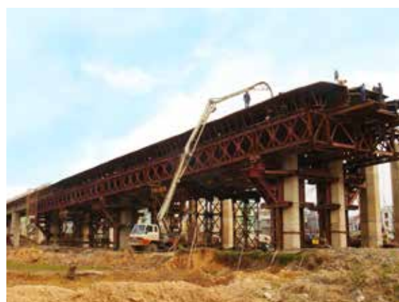
Construction of girder for BC3 Bai Chay project
