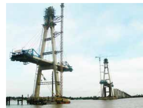
Construction of cantilever for Rach Mieu Bridge
