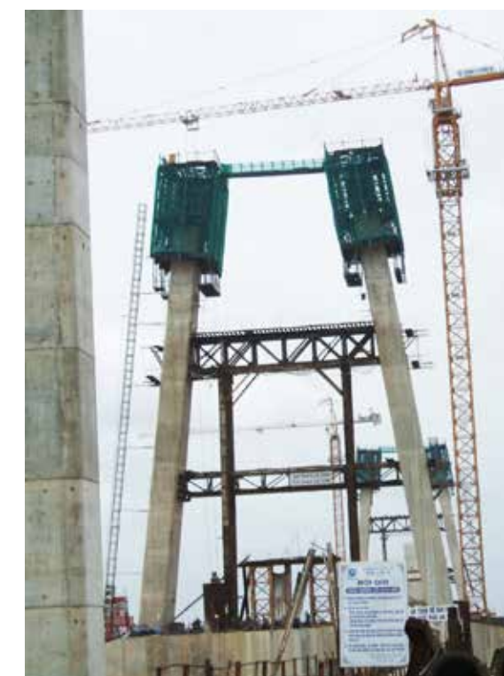
Formwork for the construction of Rach Mieu Bridge abutment
