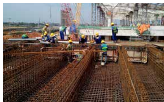
Construction of girder for Terminal T2 at Noi Bai International Airport
